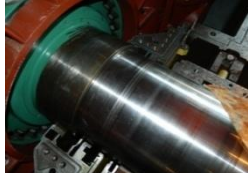
GENERATOR ROTOR SHAFT 500 MM DIA.
